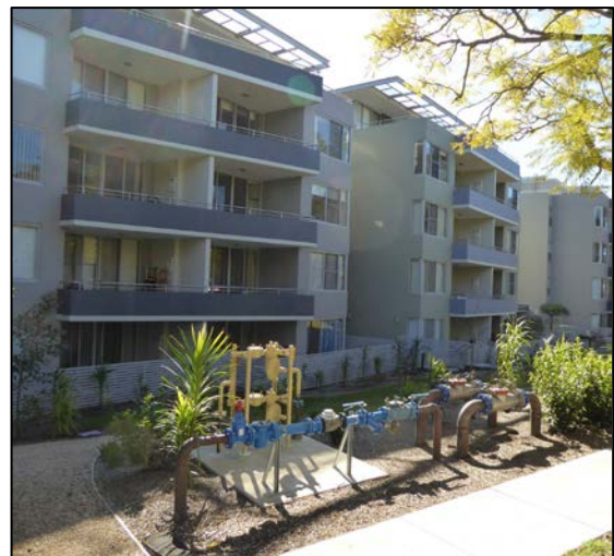
FIGURE 17: 3-7 LORNE AVENUE, NEW APARTMENT COMPLEX (SOURCE: CURIO 2016)
